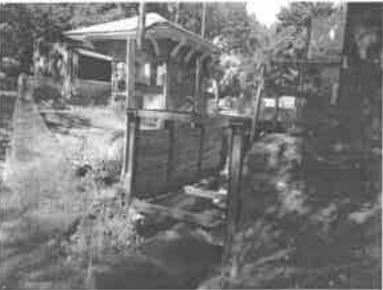
Photo 3. Shored excavation between pump house and lift station.
