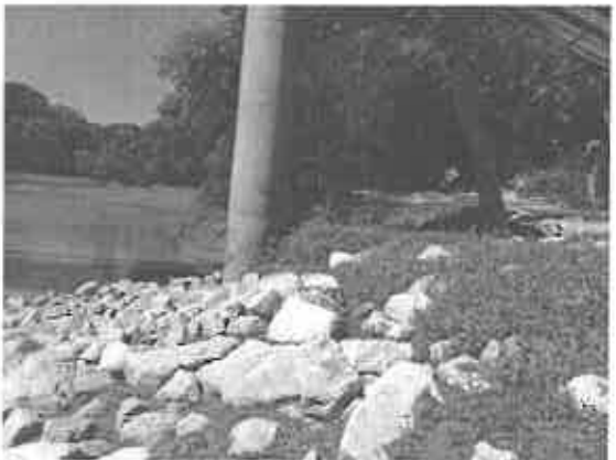
Photo 6. Riprap erosion protection. Looking upstream from downstream extent of site.
